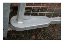
Ensure that the gate posts are set vertial and that the closing gap is constant, it must not be below 25mm.
