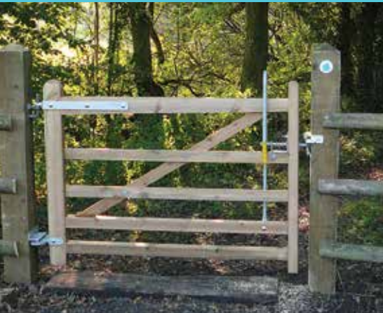
Installed Height 1200mm, o/a post to post 2100mm, Gate leaf 1600mm wide x 1200mm high
